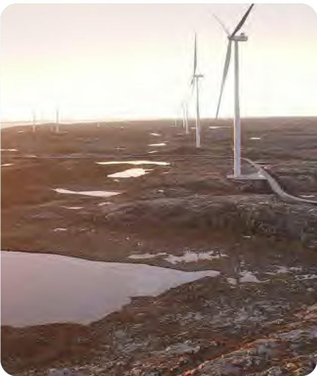
Frøya wind power plant
